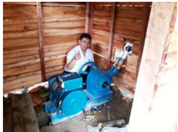
Gambar 3. Turbin Cross Flow Multi Nozzle
