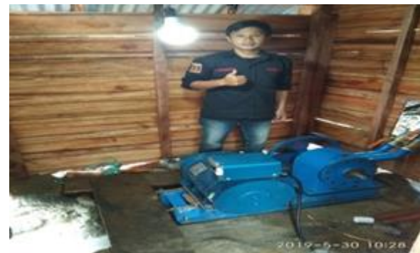
Figure-2. Installation Power Plant Produced Electric
