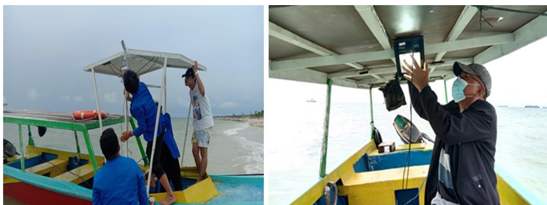
Figure 1 Installing a Solar Electric Generator on a Fishing Boat
